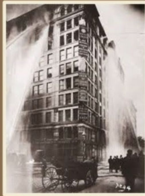
The 1911 Triangle Shirtwaist Factory fire in New York City killed 146 garment workers and helped pave the way for the Grand Bargain.
